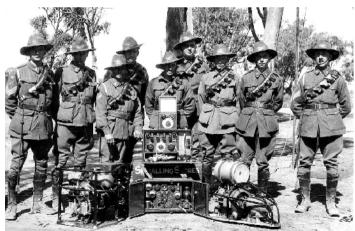
NCOs and Signalmen from 3<sup>rd</sup> Divisional Signals, Australia, 1931. The engine driven generator set at the left is a Power Unit 180 watt Mk.I driven by a Douglas engine and at the right Power Unit 180 watt Mk.II driven by a Stuart Turner engine. Note a Wavemeter C Mk.I on top of the Reception Set C Mk.II
